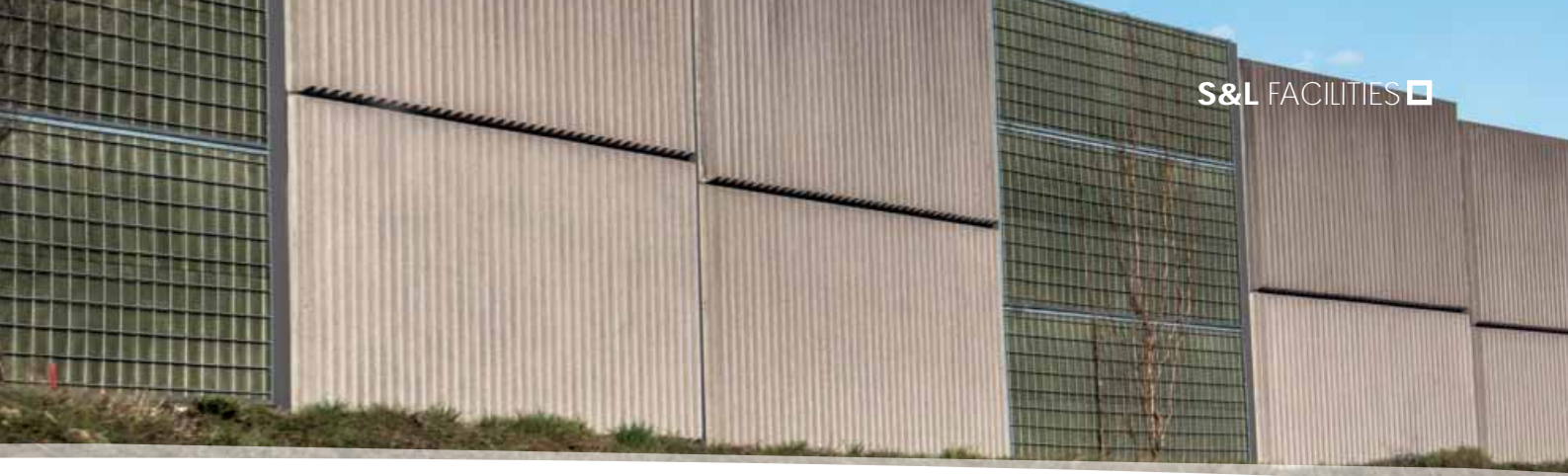
9 Foto oben: Lärmschutzwand Beton, Noise barrier made of concrete (© focus finder)
